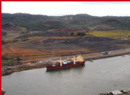
Paradise Hill, in front of the Pedro Miguel locks, has been reduced in height from 136 to 46 metres. The elevation is equivalent to a 30-storey building.
