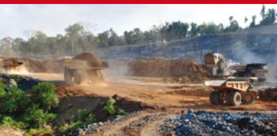
Three of the four dry excavation contracts are now in the process of being carried out.
